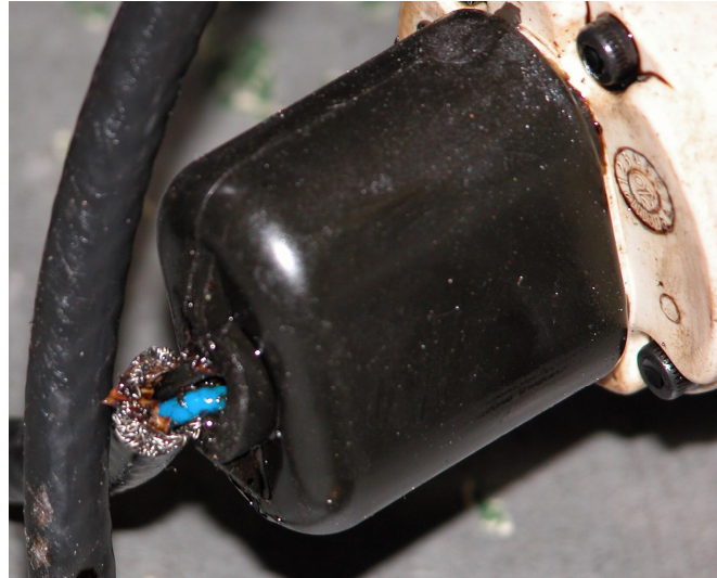
Figure 6 - Backshell destroyed by chemicals
